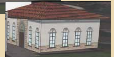
New Fourth Grade Classroom Projected Completion June 2018
